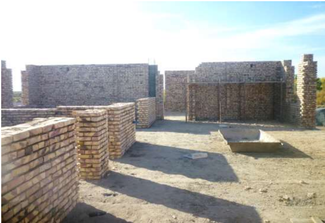
Figure 68. Construction works at Muynak biostation (September-October, 2023)
