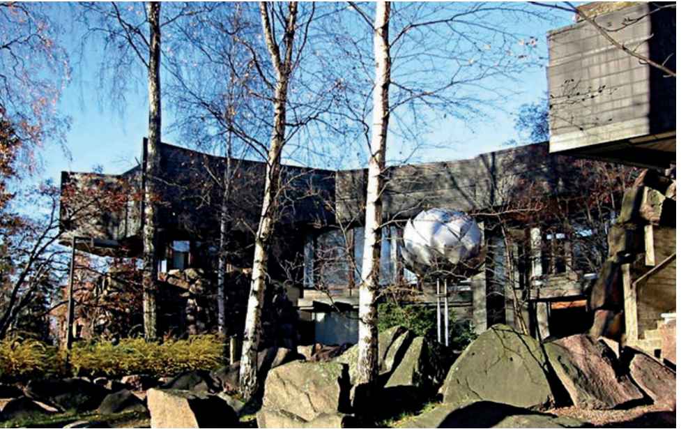
10. Side view of the Dipoli multi-functional Conference Center situated on the campus of the Helsinki University of Technology on the Otaniemi peninsula in Espoo, located some 9 kilometers North-West of Helsinki.
