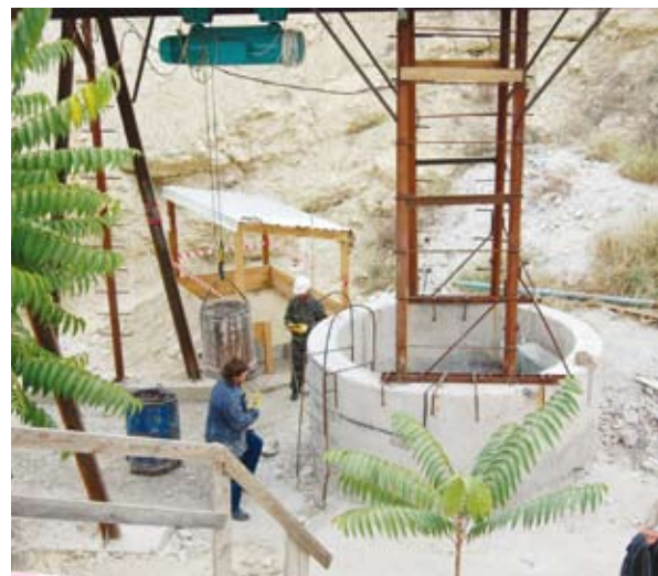
Inkerman Caves. These mountainside entrances to the former ammunition warehouse of the Soviet Black Sea Fleet are still in use, but several collapsed and were blocked after a World War II explosion. The Ukrainian Government is constructing shafts to gain access to collapsed caves. (OSCE/Niels Poul Petersen)
