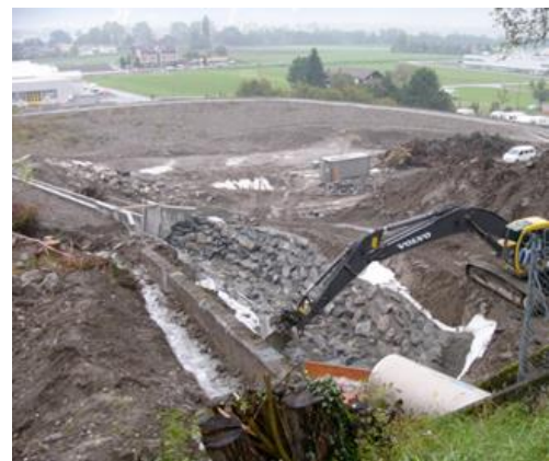
Figure 17: Construction of the retention basin in 2003.
