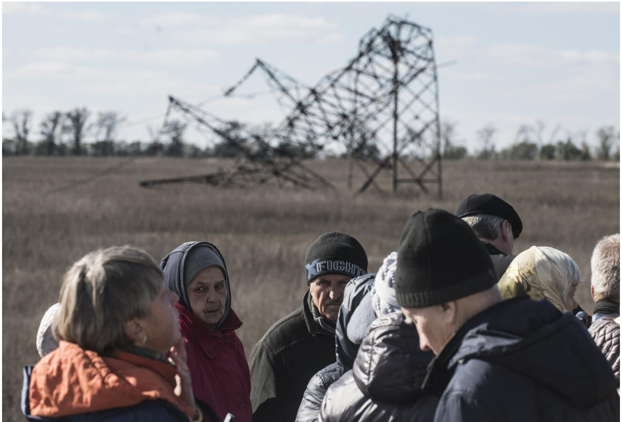
Figure 4: Civilians near damaged power lines close to Marinka, 2016.
